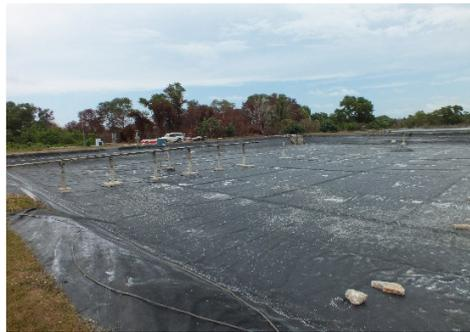
*HDPE liner pond for prevention of Acid Sulfate Soil contamination of soluble iron which caused slow growth and mortality during raining seasons.*
